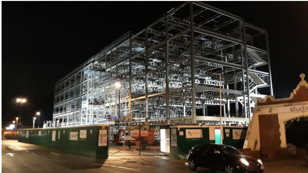
Teville Gate House Construction 12/12/2019
